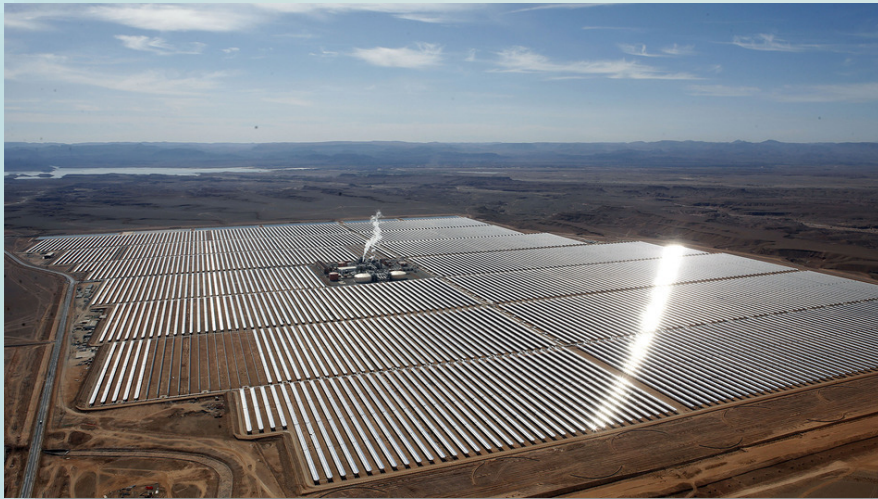
Morocco: Noor I, production volume of 160 MW
