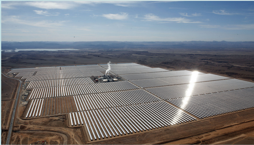
Morocco: Noor I, production volume of 160 MW
