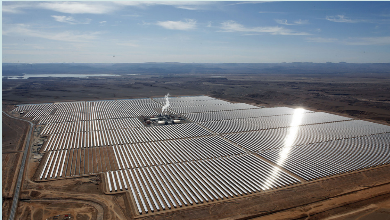
Morocco: Noor I, production volume of 160 MV
